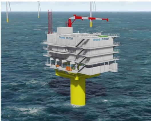
***Atlantique Offshore Energy, Chantiers de l'Atlantique's Business Unit dedicated to Marine Energy, has been selected by Ørsted to execute the full Engineering, Procurement, Construction and Commissioning of the Electrical Offshore Substation (Topside and Modular Support Frame) required for the Gode Wind 3 Offshore Windfarm, to be installed in 2023 in the German North Sea.***
